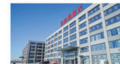
Intelligent comprehensive production base
