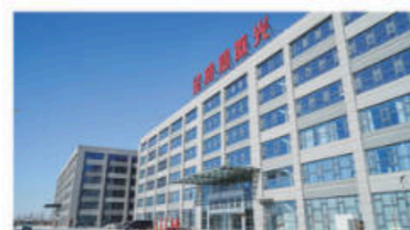
Intelligent comprehensive production base
