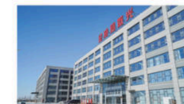
Intelligent comprehensive production base
